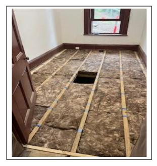
With help from David Pryor and the rest of the Property Committee this has been a frustrating and demanding project. A plumber was engaged to install a drainage system along the side, even the downpipes outside the kitchen extension had not been connected. During this wet winter, water has poured through the foundations. Termites love water!
